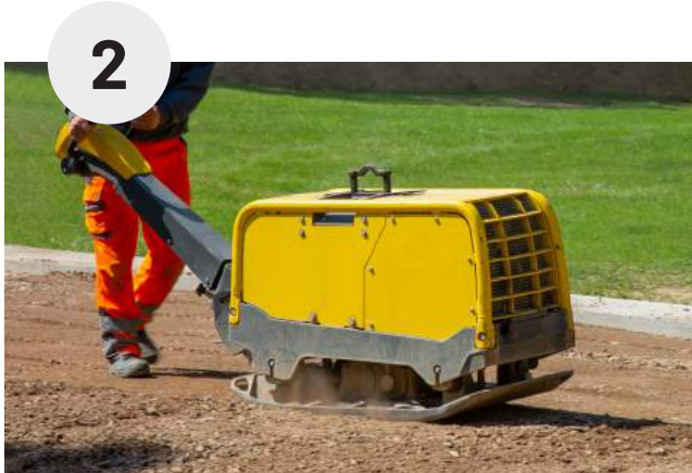
Lu nén nền | Compaction of the ground
