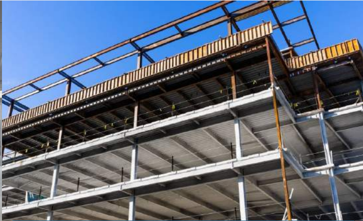
Sàn Deck Deck Floor
