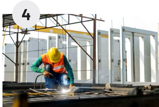
Lắp đặt joint | Installing joints
